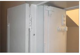
The outer and inner doors of the Burke's Building vault, of Pittsburgh steel, are secured by a keyed lock, not a combination, as reported in some accounts of the Denny Estate theft. Photo by Tim Bintrim.
