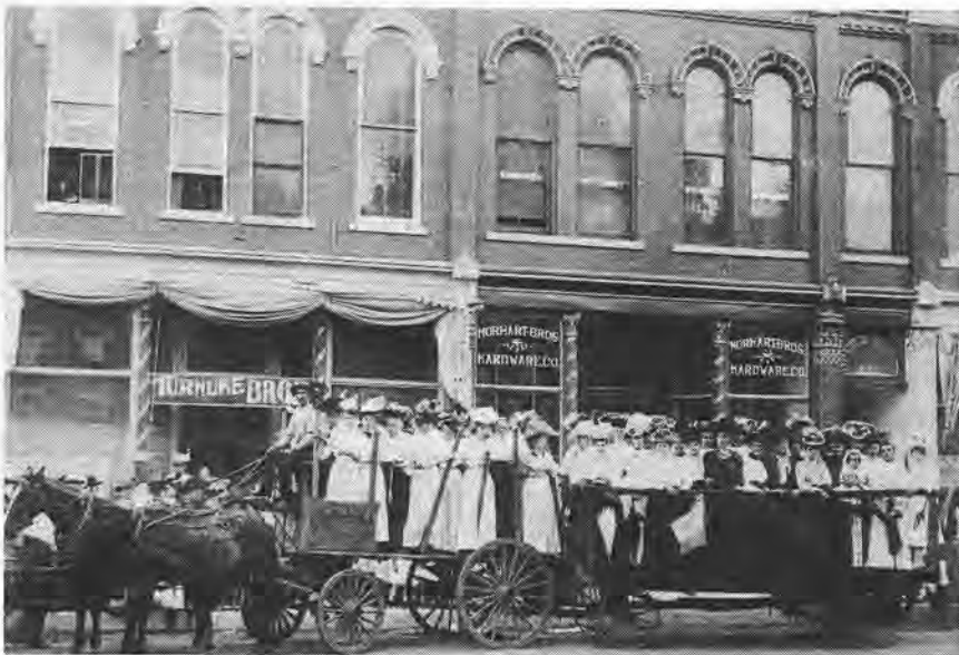
Undated photograph of the south side of the 1885 Opera House. The moon-shaped window on the far right side is above the entrance leading upstairs to the Opera House. The north half of the Opera House is not shown.
