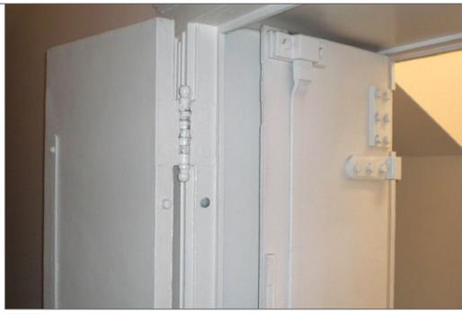
*The outer and inner doors of the Burke's Building vault, of Pittsburgh steel, are secured by a keyed lock, not a combination, as reported in some accounts of the Denny Estate theft. Photo by Tim Bintrim.*
